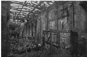
FIG. 2. An illustration of some of the damage caused by the fire in St. George's Hall.
