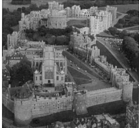
FIG. 1. Windsor Castle: a view of the present Castle looking east.
